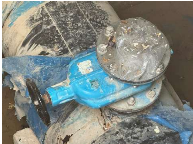
Gate valve entry point
