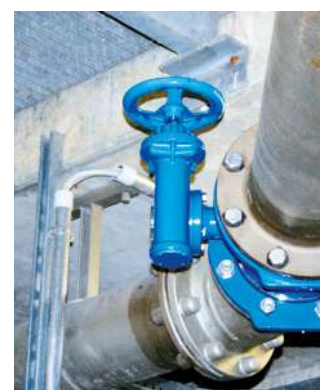
The valve can be turned after installation into its final position.
