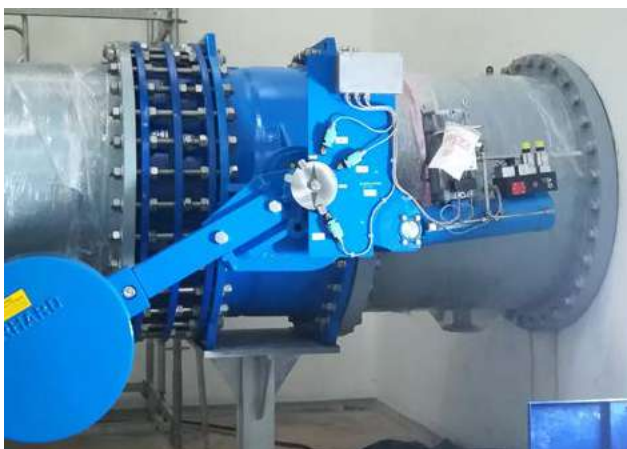
Standard: 3 limit switches for "open", "closed" and "90% open"
